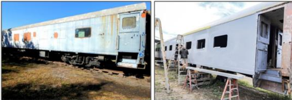
Side Away from the Building
